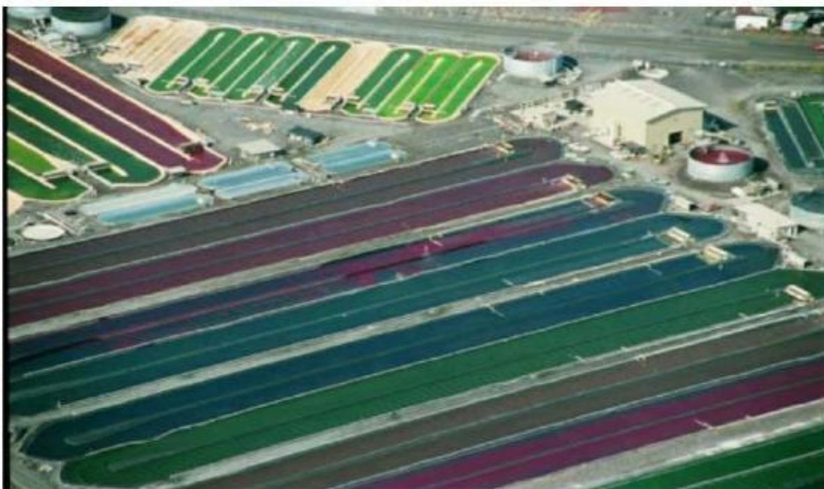
Cyanotech Corporation natural Haematococcus algae astaxanthin production facility in Kailua-Kona, Hawaii. The large ponds hold approximately 500 cubic meters of algal culture.
